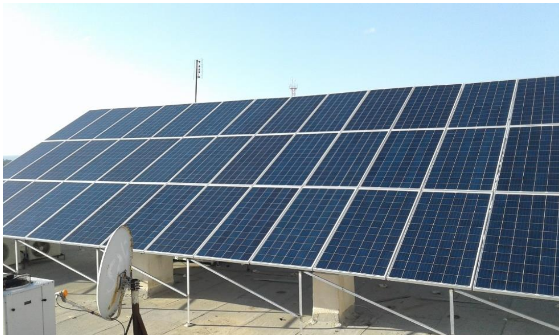
Figure 16: Solar Panels on the top of Al Aqsa Hospital
