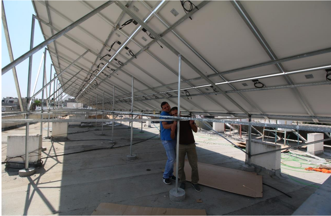
Figure 23: Checking the Steel Structure of the Solar Panels in Beit Hanoun Hospital
