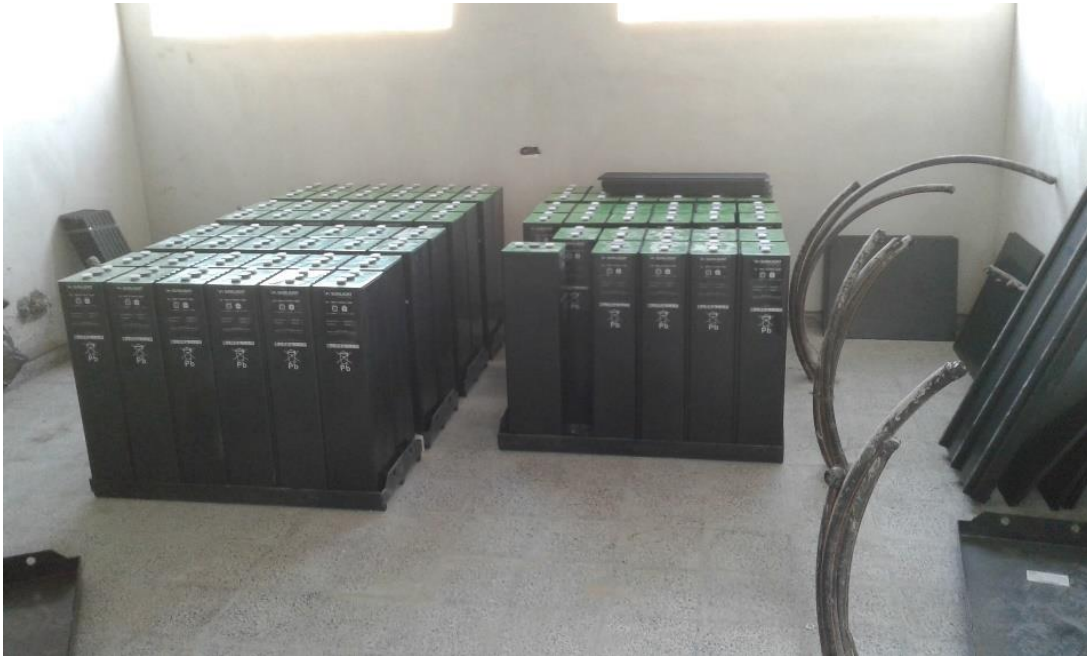
Figure 7: Supplied batteries in the Batteries Room at Indonesian Hospital
