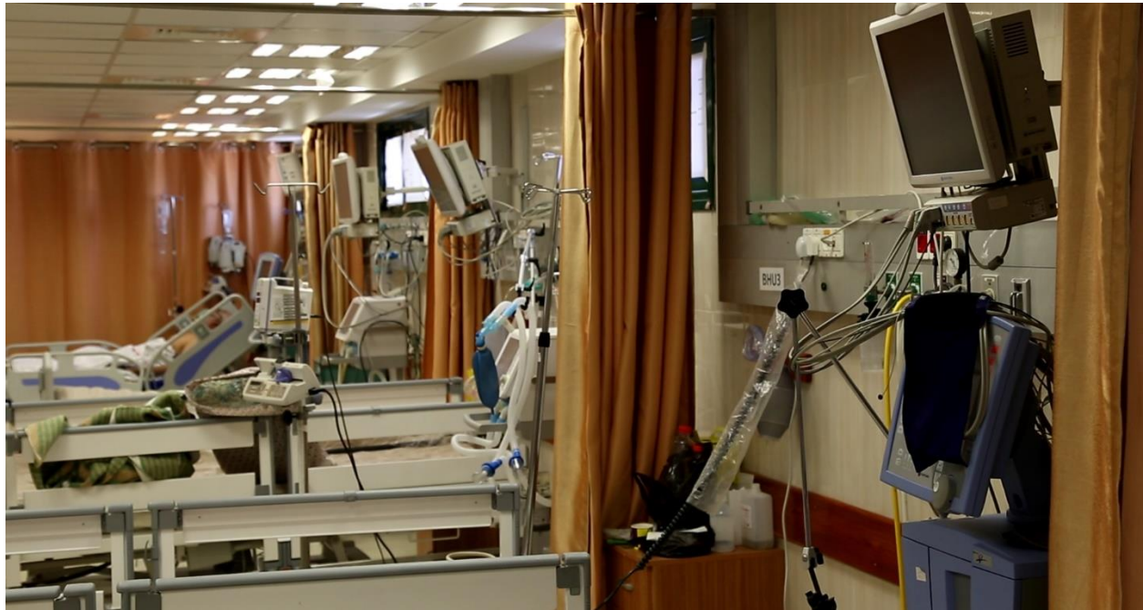
Figure 13: ICU powered by Solar Energy - Al Aqsa Hospital
