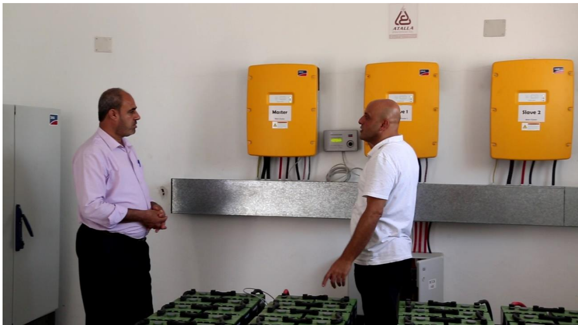
Figure 22: Guidance given to Hospital Administrator on the Operation of the Solar System at Beit Hanoun Hospital
