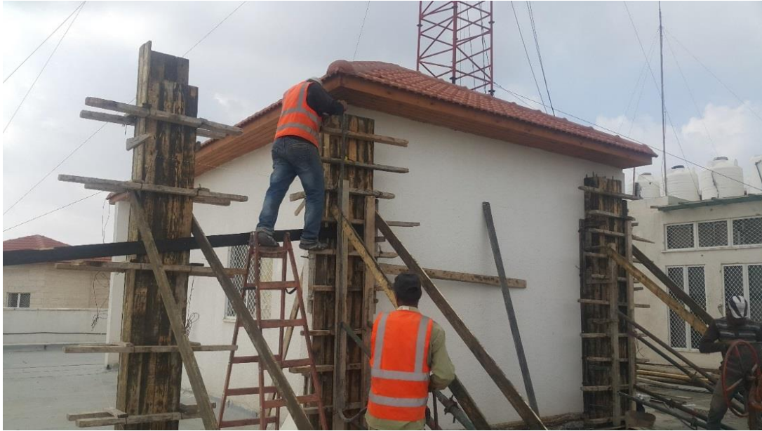
Figure 5: Construction of the Batteries Room on the top of the Indonesian Hospital
