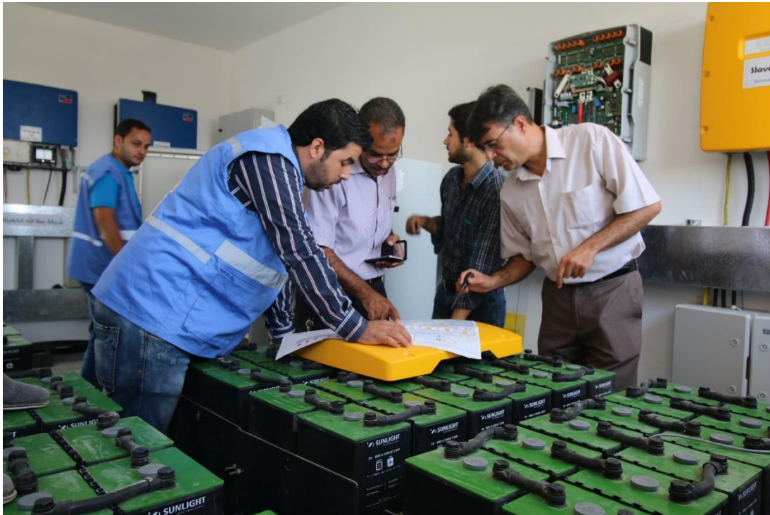
Figure 15: Testing the installation of Solar System in Al Aqsa Hospital
