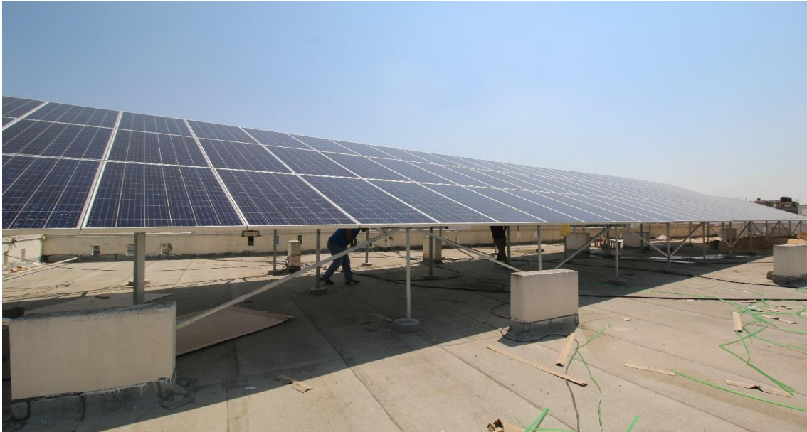
Figure 17: Solar Panels installed on the top of Beit Hanoun Hospital
