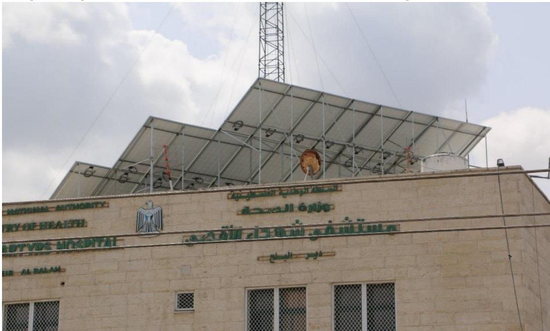
Figure 8: Solar Panels on the top of Al Aqsa Hospital in Deir El Balah
