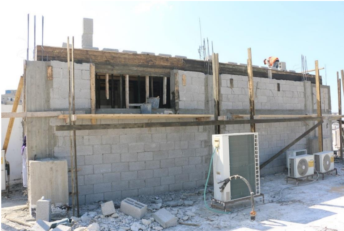
Figure 6: Construction of the Batteries Room on the top of the Indonesian Hospital
