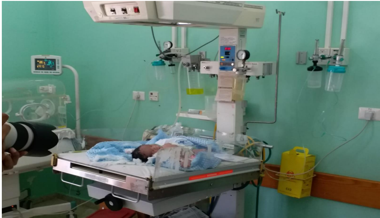
Figure 11: Nursery Unit powered by Solar Energy - Al Aqsa Hospital
